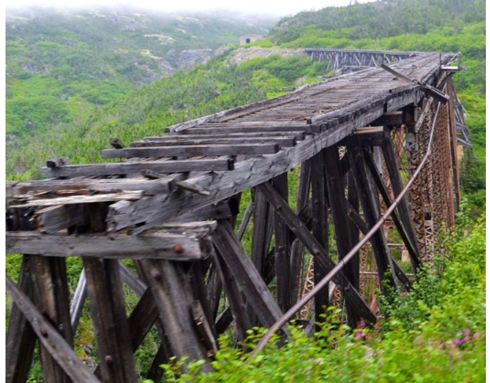
White Pass - Not On This Bridge!
