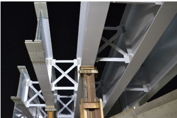
3. Rte. 72 Bridge Superstructure
