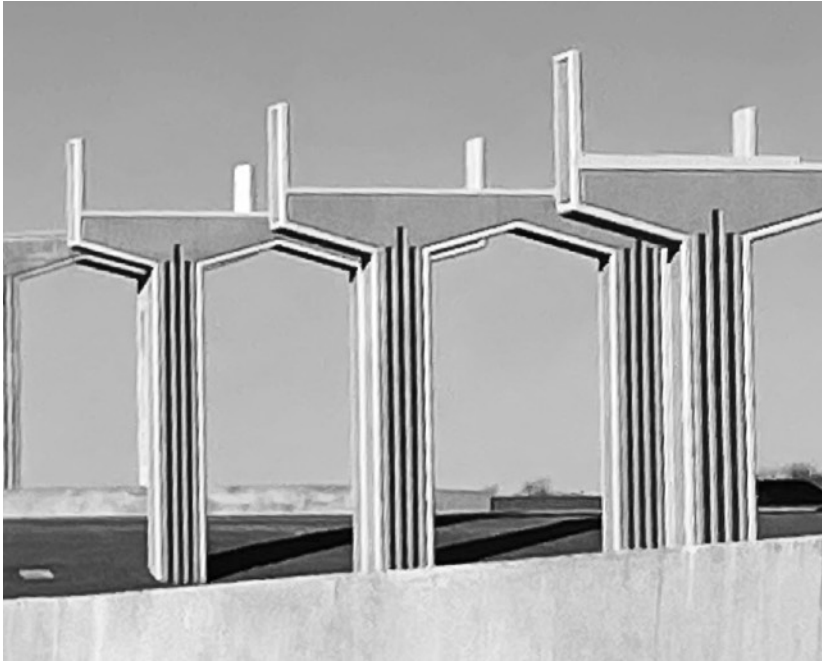
1. A Group of Piers Waiting for Their Beams
